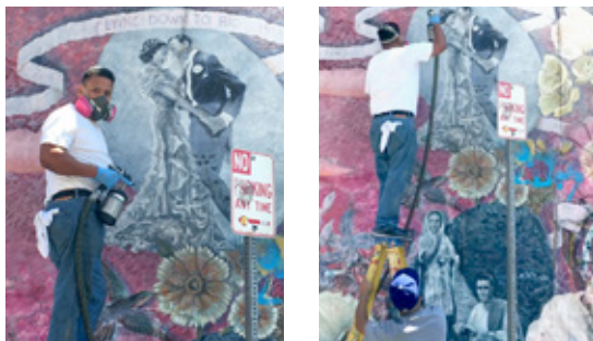
MURALSHIELD being applied with HVLP sprayer
